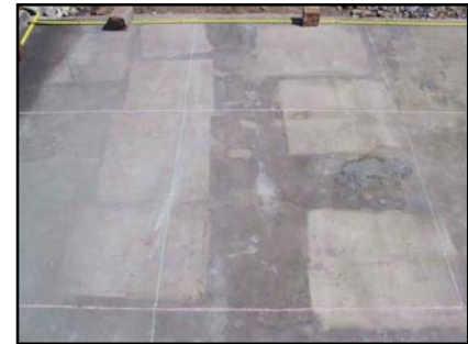
Figure 10: Impressions, made by the fire, of stored items were found on the concrete slab once all remains had been cleared.
